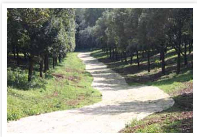
The gully restored following damage created by soil erosion
