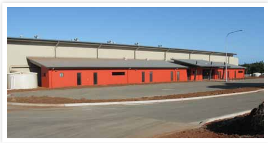
The new Bundaberg factory progressing well with fit-out underway
